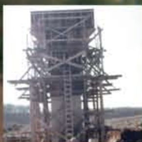
Building the infrastructure underneath Lake Anne
